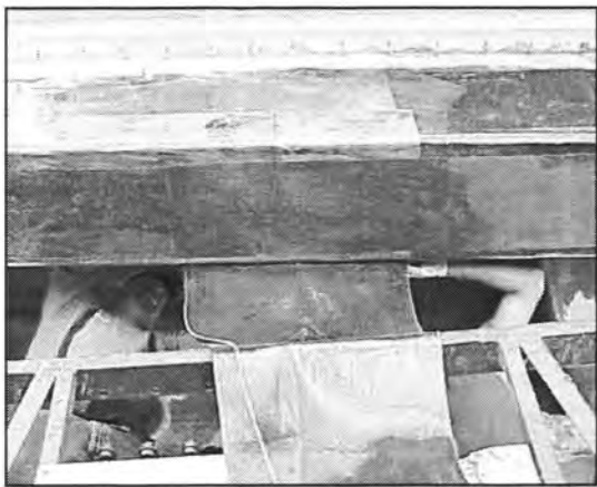
Figure A18. Transverse wrap over the longitudinal FRP.
