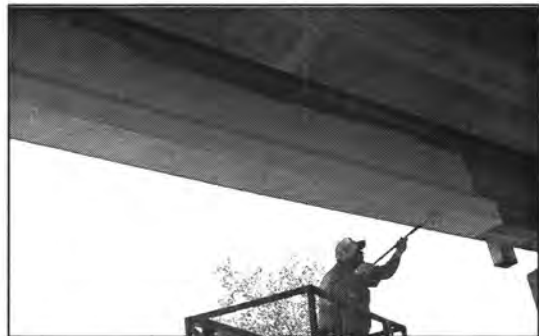
Figure A22. Using a roller to paint bottom flange.
