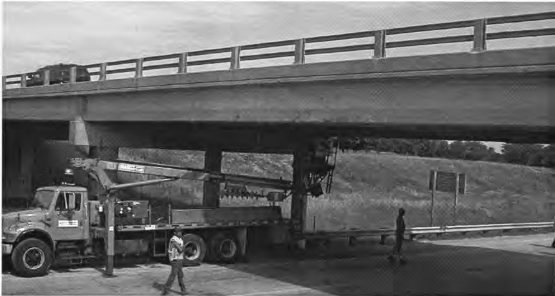
Figure 3.37. Overall view of De Soto Bridge looking southeast.
