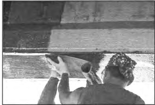
Figure A17. Four inch overlap splice.
