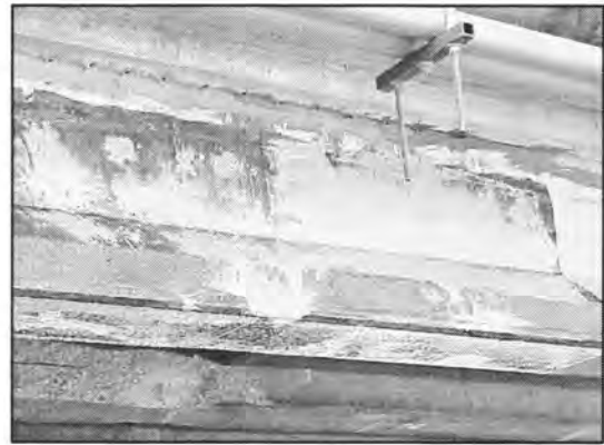
Figure A10. View with putty step completed.
