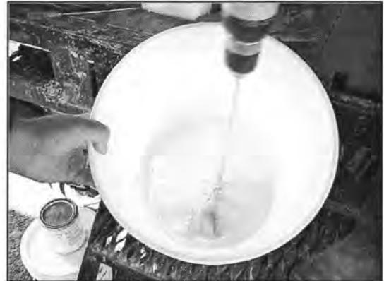
Figure A4. Mixing of the primer components with mixing drill bit.
