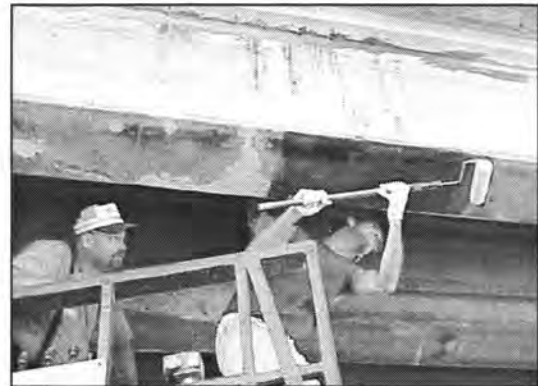
Figure A6. Another view of primer application.
