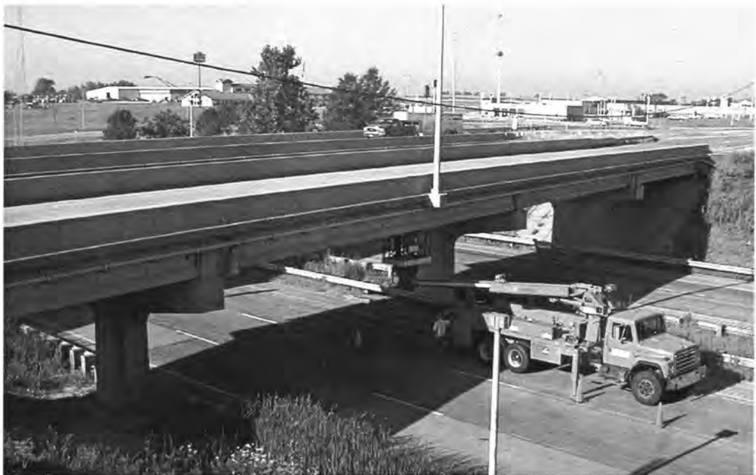
Figure 3.28. Overall view of the Osceola Bridge looking southwest.
