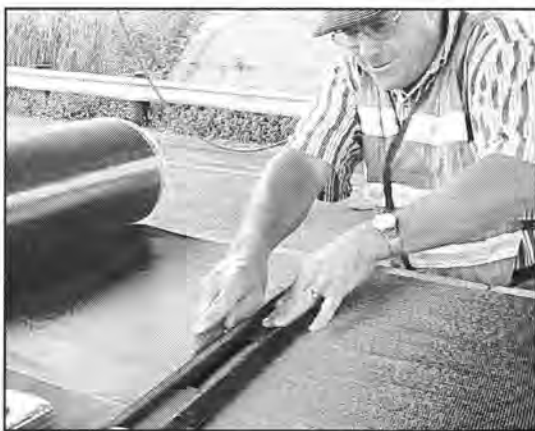
Figure A14. Cutting FRP to the predetermined size.
