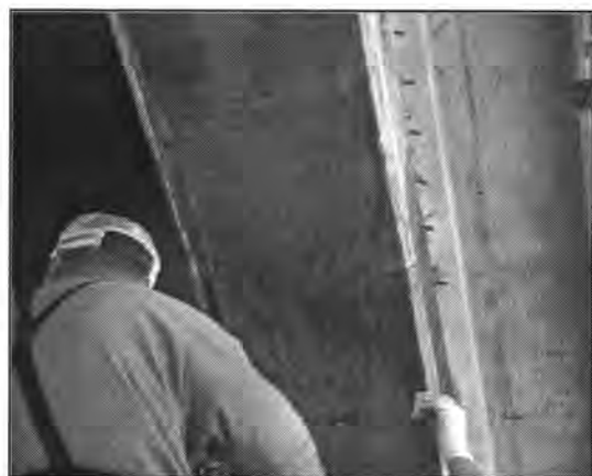
Figure A15. One strip of longitudinal FRP.
