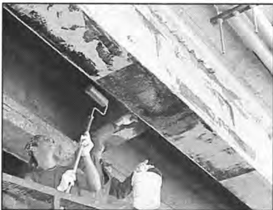
Figure A13. Applying saturant.
