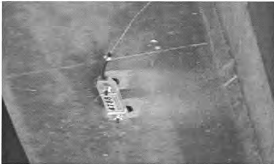
Figure 3.33. Close-up of BDI gage on the Osceola bridge.
