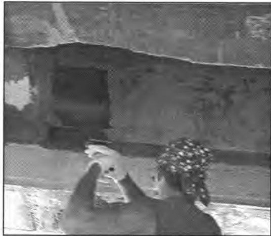
Figure A12. Beginning the application of saturant layer with nap roller.
