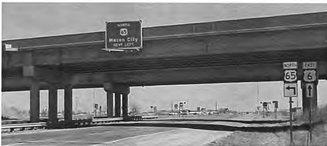
Figure 3.16. Overall view of Altoona Bridge looking east.
