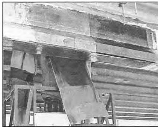
Figure A19. Transverse wrap (cut to designed length).
