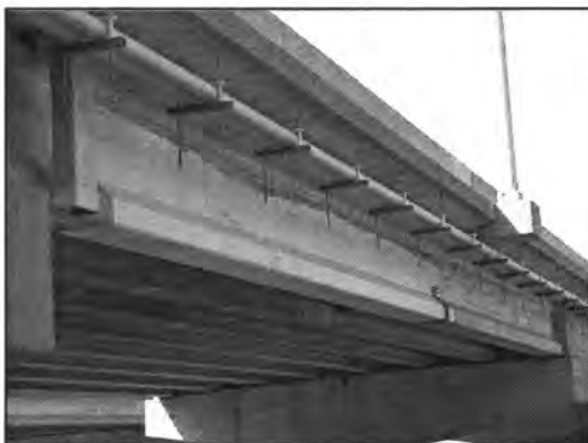
Figure A23. Final view of completely repaired bridge.
