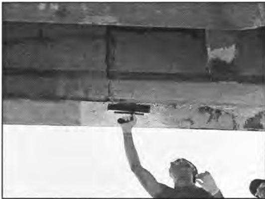
Figure A9. Applying putty with hand trowel.
