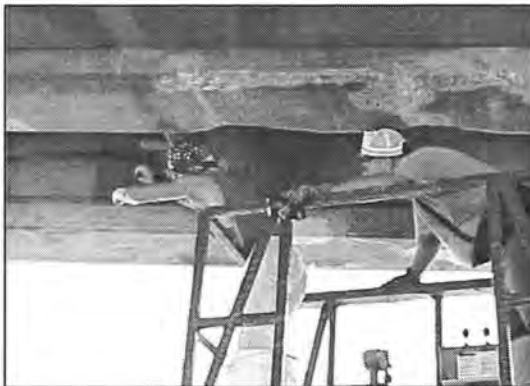
Figure A5. Applying primer with nap roller.
